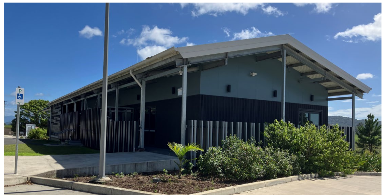
Stotts Creek Resource Recovery Centre Offices and Training/Education Room
