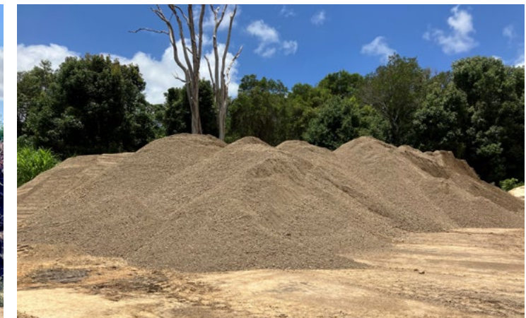
Recovered aggregate to be used in road construction
